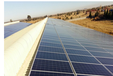
Rooftop structure with PowAR® Snap - SOUTH AFRICA
